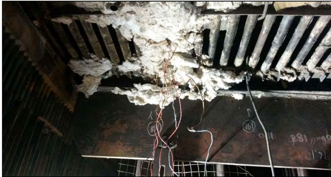
Figure B4.6: PWHT in progress
